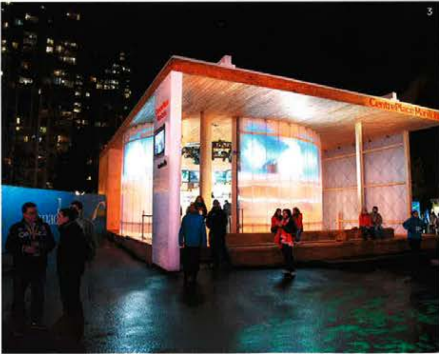
LIGHT SPILLS FROM THE MULTIMEDIA DISPLAY WITHIN THE PAVILION, THROUGH THE TRANSLUCENT WALLS TO THE EXTERIOR, ELIMINATING THE NEED FOR SITE LIGHTING [3].
