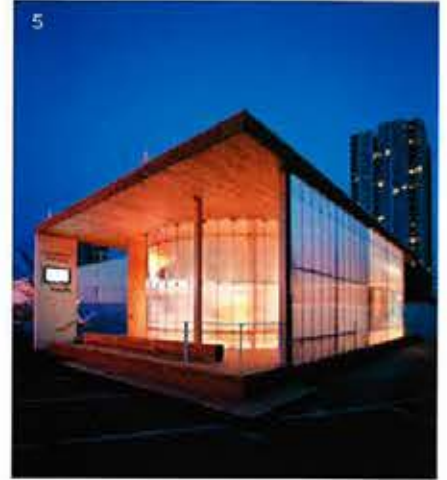
SPACED BOARDS ON THE FLOOR AND CEILING, TOGETHER WITH AN OVERSIZED PIVOTING DOOR ENABLED THE PAVILION TO BE NATURALLY VENTILATED [4]. THE PAVILION GLOWS LIKE A WELCOMING LANTERN ON ITS PARKING LOT SITE IN DOWNTOWN VANCOUVER [5].
