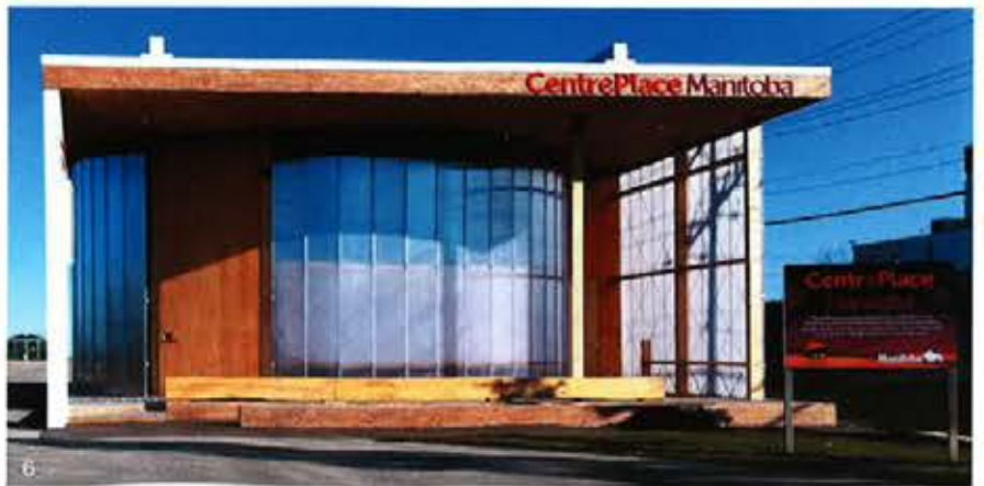
DISMANTLED AFTER THE OLYMPICS, CENTRE PLACE HAS NOW BEEN RELOCATED TO THE RED RIVER EXHIBITION GROUNDS IN WINNIPEG [6].
