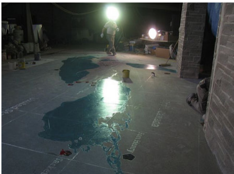
After terrazzo is poured
