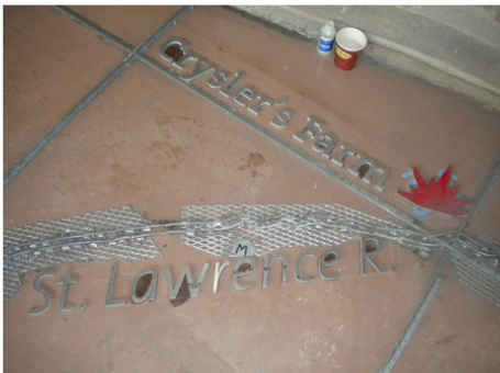
3D letters and the outlines of the map are in position before the terrazzo are poured in
